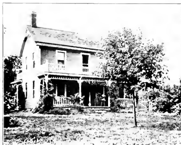
MAJOR WILSON'S RESIDENCE
