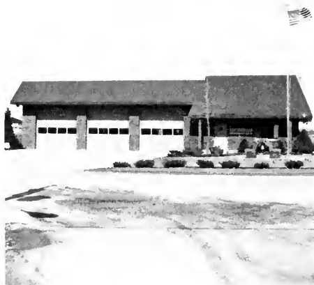
New Fire Station
