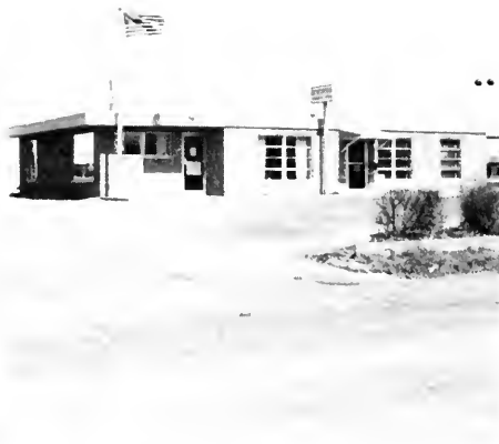
Limestone Township Hall
