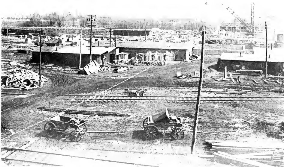
Keystone's Steel Mill under construction in 1917
