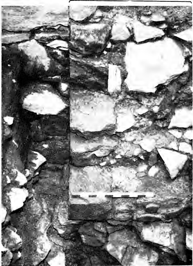
Trench C/2. Showing the three phases of wall and the possible buttress.
