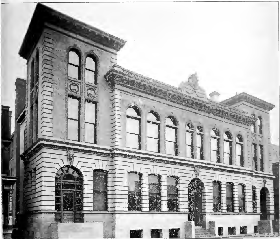
High School Building, Seventh Avenue between Fourteenth and Fifteenth Streets, Altoona, Pa.
