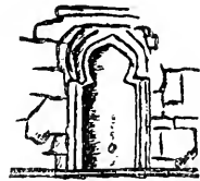
PORCH NICHE, CALSTONE CHURCH.
