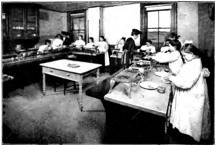
CHILDREN'S ROOM AND KITCHEN, CHRIST CHURCH MEMORIAL HOUSE
