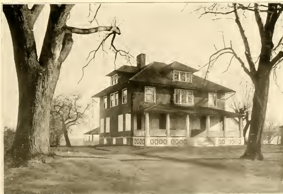
FAIRFIELD FRESH AIR HOME FOR CHILDREN
