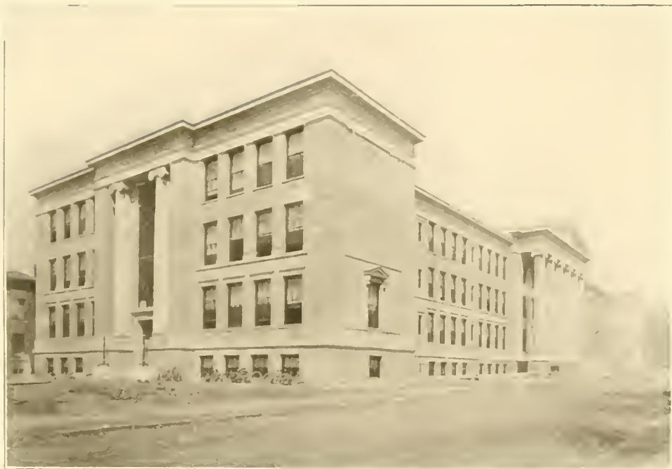
NEW HIGH SCHOOL BUILDING, BRIDGEPORT
