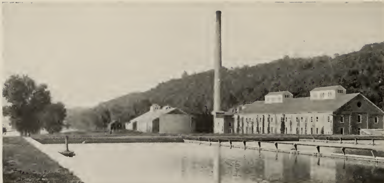
WATER-WORKS PUMPING STATION
