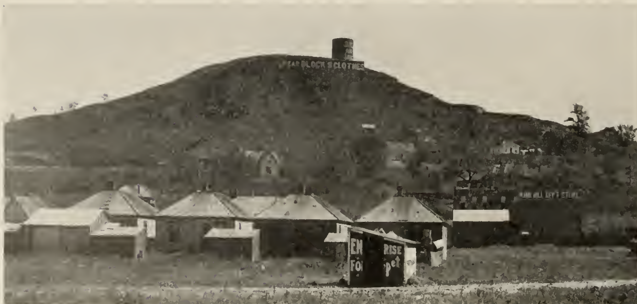
VIEW OF KING HILL, SOUTH ST. JOSEPH (Showing Stand-Pipe from Which South St. Joseph Draws Its Water Supply)
