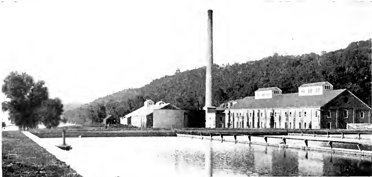
WATER-WORKS PUMPING STATION
