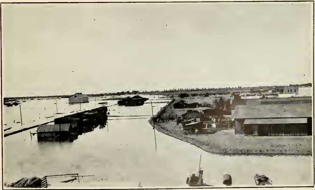
Flood scene showing the levee.
