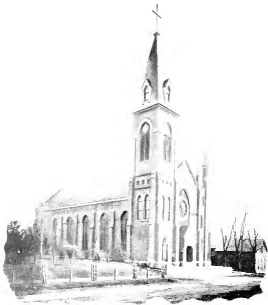
ST. MARY'S CHURCH, GREENSBURG, IND.
