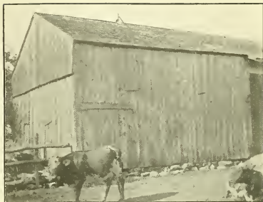
FIRST FRAME BARN ERECTED IN SHERIDAN.
