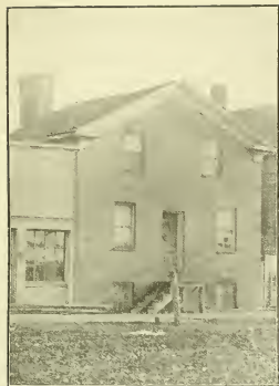
SAMPSON ALTON'S HOUSE, DUNKIRK First Brick House in Chautauqua County
