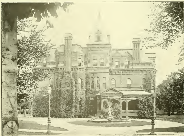
BROOKS MEMORIAL HOSPITAL AND LIBRARY BUILDING, DUNKIRK, N. Y.
