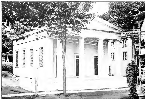
GRANGE BUILDING, CHAUMONT
