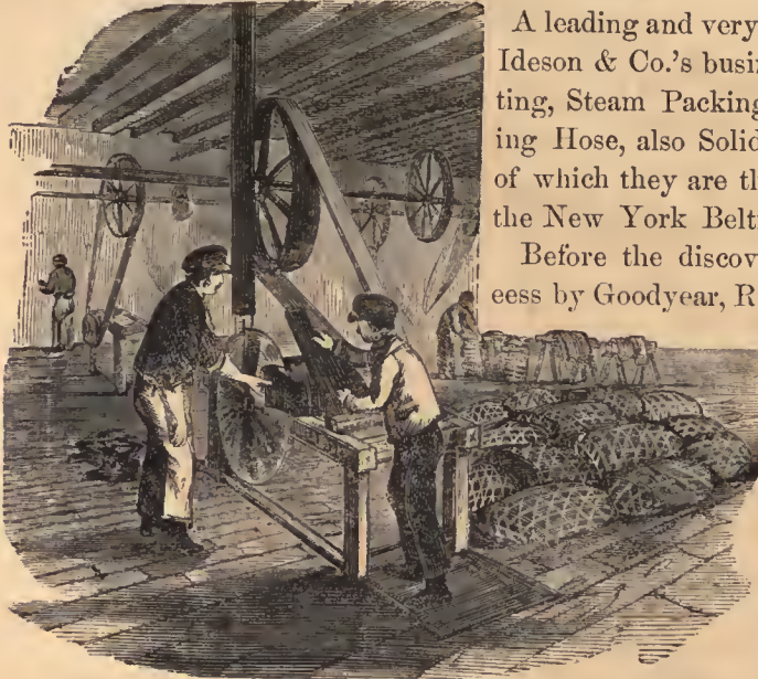
CUTTING RUBBER INTO SLABS FOR THE WASHROOM.
