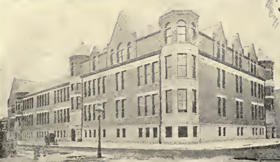
NORTH-WEST DAWSON HIGH SCHOOL NORTH-EAST CORNER OF SEABY STREET AND POTOMAC AVENUE
