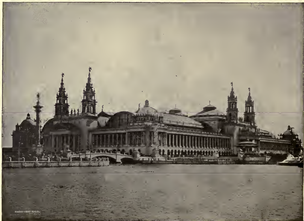
MACHINERY HALL. Size, 846 by 492 feet. Floor area, 17½ acres. Annex, 550 by 490 feet. Floor area of Annex, 6 acres. Cost, $1,200,000.
