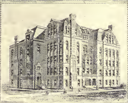
ANDERSEN SCHOOL BUILDING Location School near Division Street
