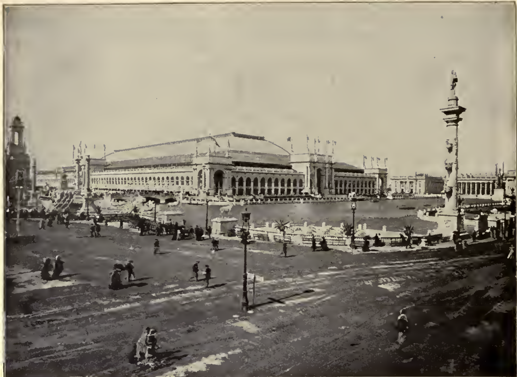
MANUFACTURES BUILDING FROM MACHINERY HALL. Size, 1687 by 787 feet. Covers 32 acres. 7,000,000 feet of lumber in the floor. Cost, $1,700,000 Largest building in the world. Three times larger than St. Peter's at Rome Highest point of roof, 237.6 feet.
