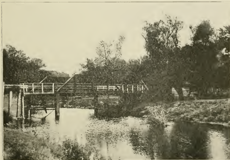
RED BRIDGE CROSSING CRANE CREEK NEAR LAWLER
