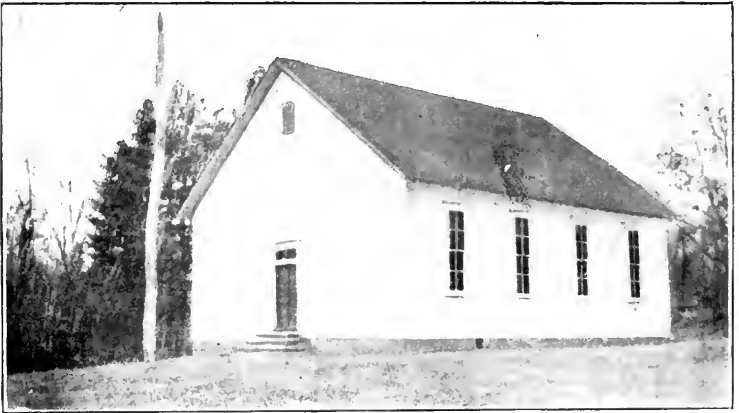
Purchase Line Church, Manor Congregation.
