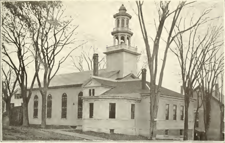
CONGREGATIONAL OR NORTH CHURCH. EXTENSION ADDED 1889
