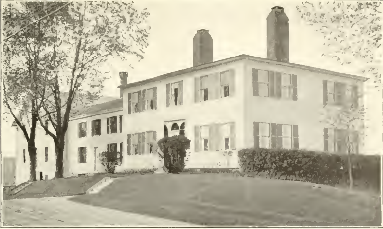
BOHAN PRENTICE FIELD HOMESTEAD. BUILT 1807
