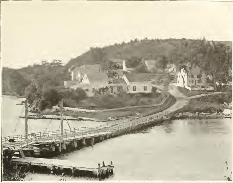
UPPER BRIDGE, PASSAGASSAWAKEAG RIVER
