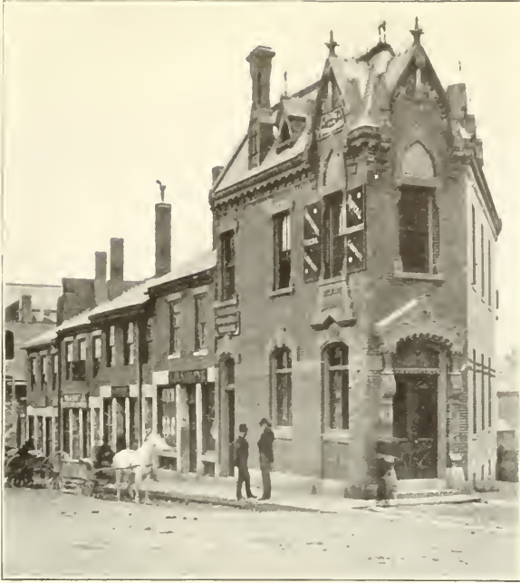
BELFAST NATIONAL BANK. ERECTED 1878
