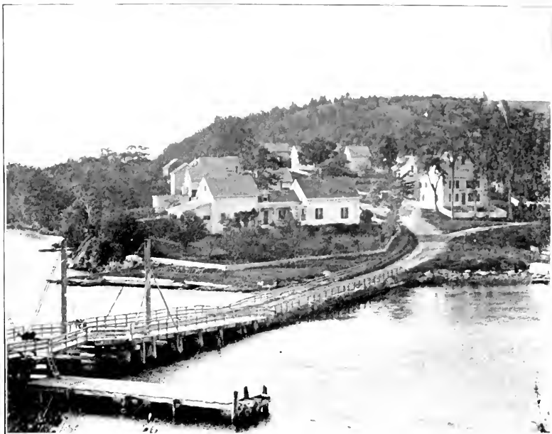
UPPER BRIDGE, PASSAGASSAWAKEAG RIVER
