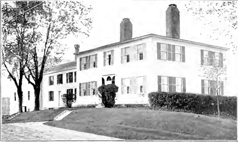
BOHAN PRENTICE FIELD HOMESTEAD. BUILT 1807
