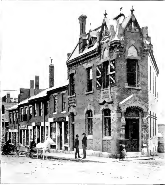
BELFAST NATIONAL BANK. ERECTED 1878
