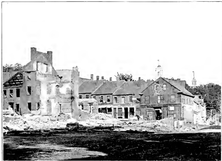
RUINS AMERICAN HOUSE FIRE, 1885
