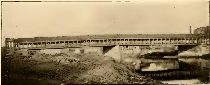
Old Broad Street Bridge over the Scioto.
