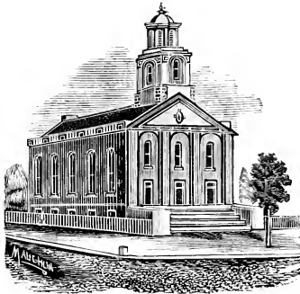
PRESENT FIRST CHURCH, BEFORE ALTERATION.
