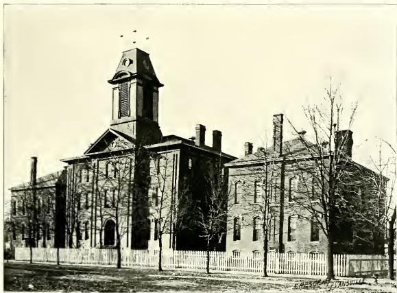
CENTENNIAL SCHOOL BUILDING
