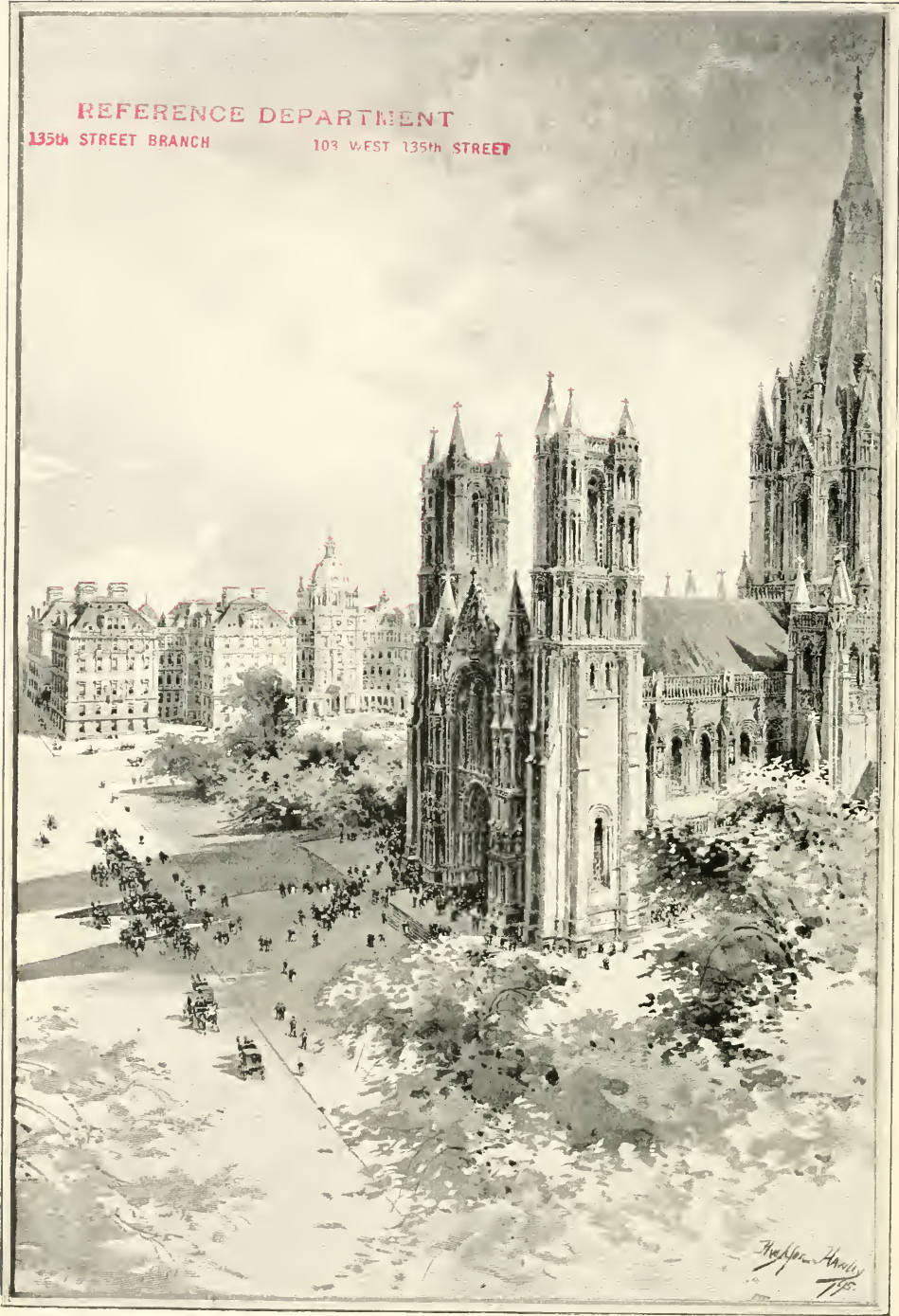
St. Luke's Hospital.
