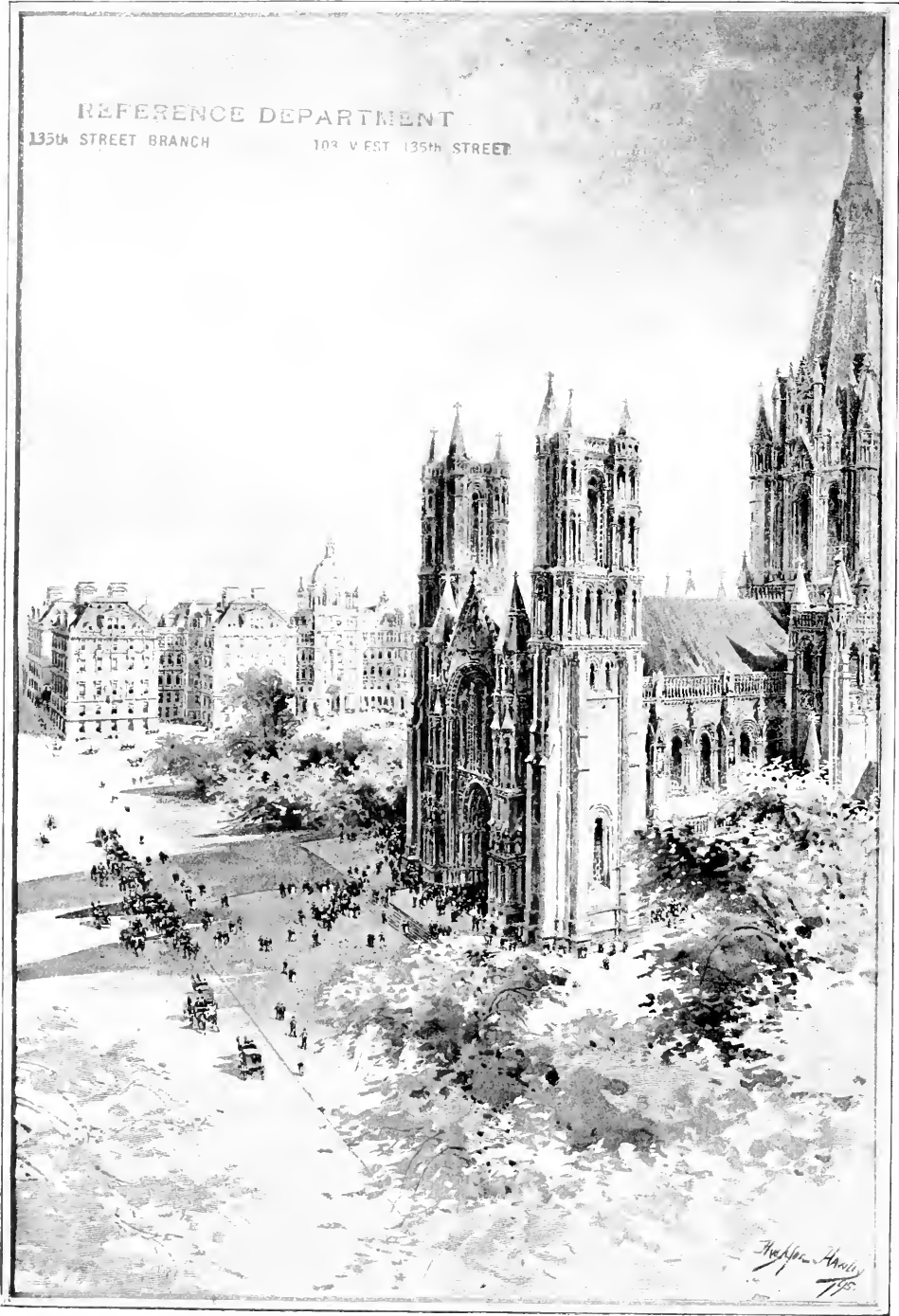
St. Luke's Hospital.
