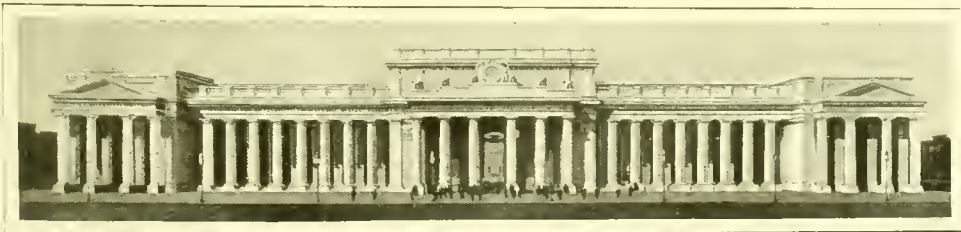
McKim, Mead & White, Architects
