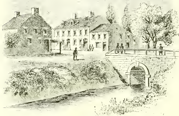
THE STONE BRIDGE, 1800 At Canal Street and Broadway
