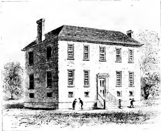
First City Poor-House.
