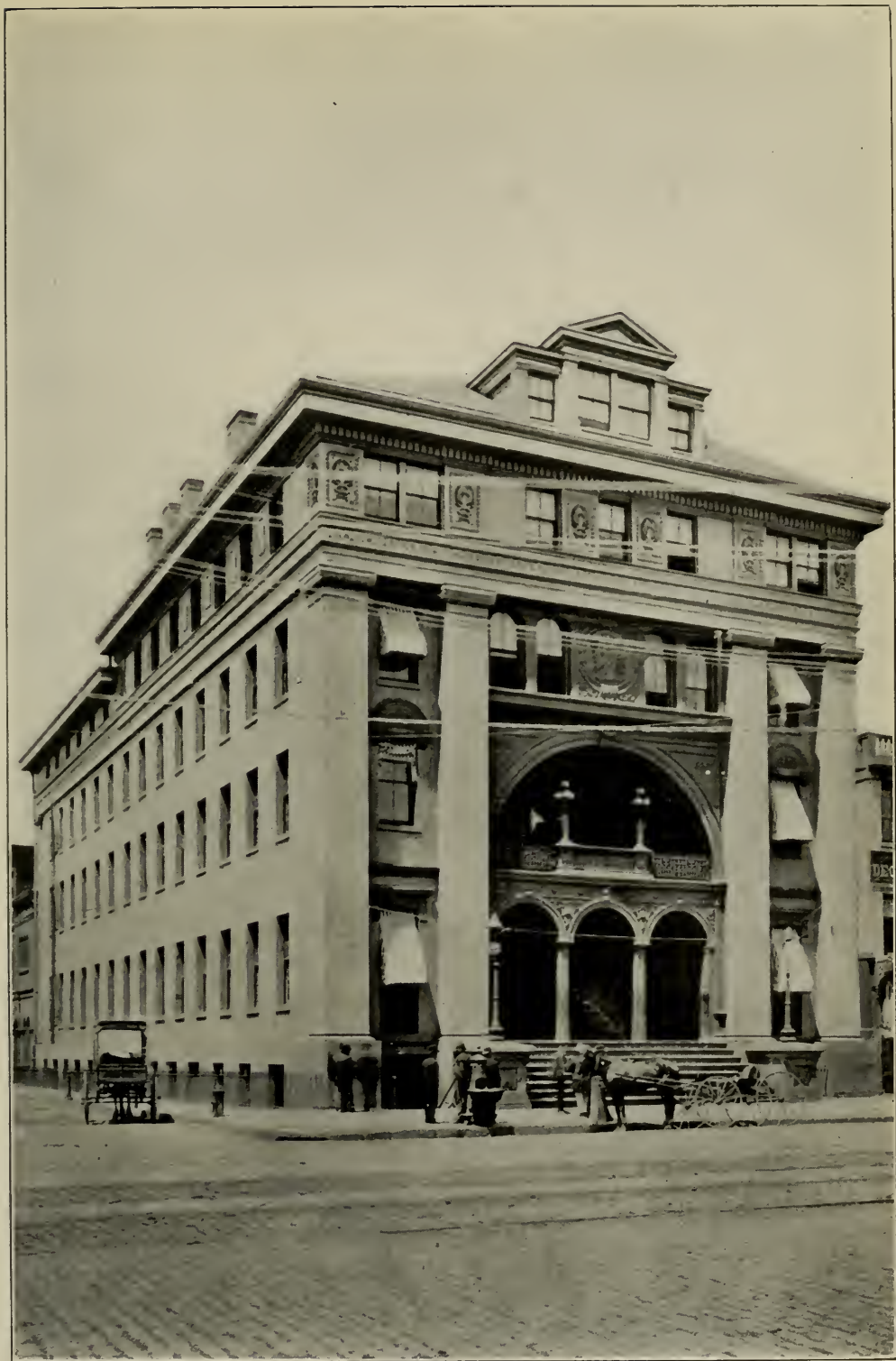
OLD CITY HALL Just before it was demolished
