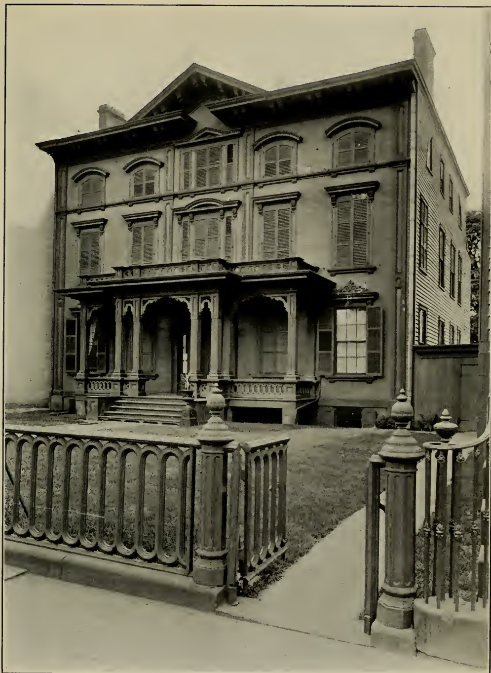
ELISHA BOUDINOT HOUSE IN PARK PLACE, 1913 Just before it was demolished
