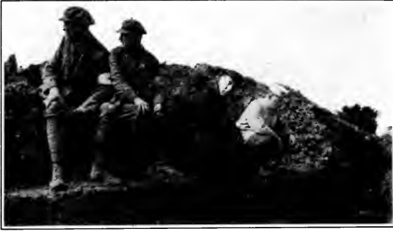
C. B. MUNSON AND COWLES IN THE TRENCHES
