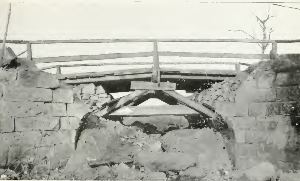
"A" TYPE BRIDGE CONSTRUCTED BY "F" COMPANY NEAR RIAVILLE,
