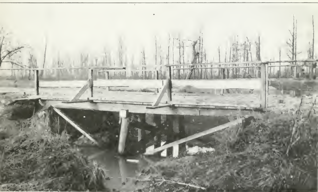
BRIDGE BUILT BY COMPANY "F" IMMEDIATELY FOLLOWING THE GRANTING OF THE ARMISTICE TO FACILITATE FOLLOWING UP OF BOCHE ARMY.
