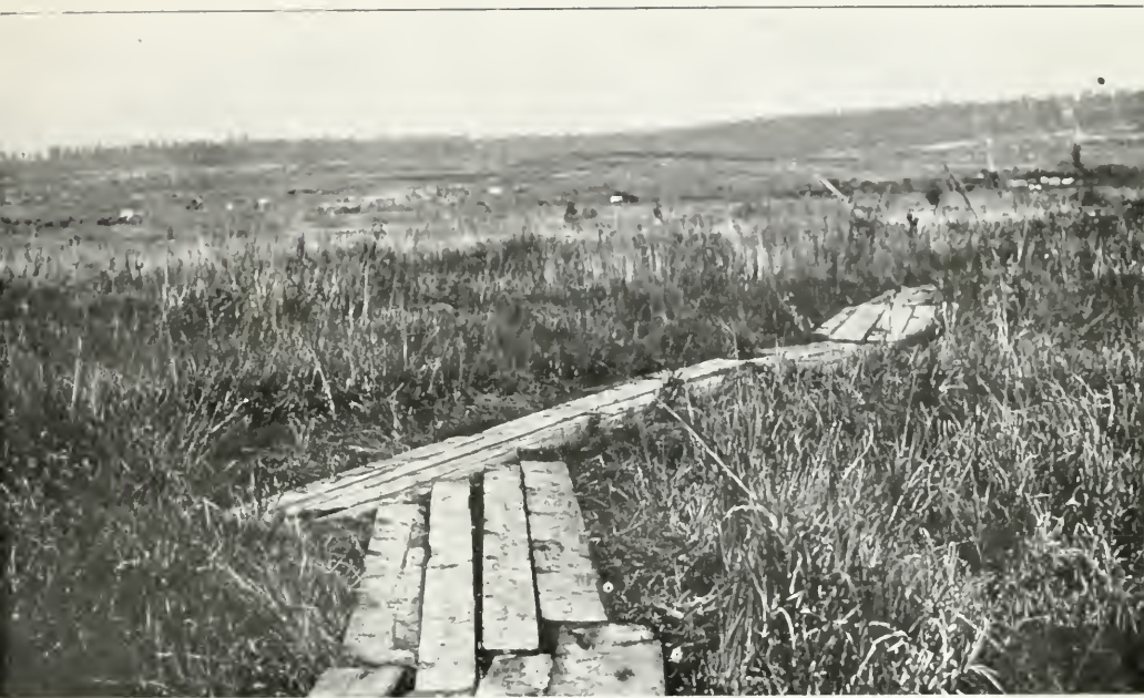
BEGINNING OF PASARELLE ACROSS FORGES SWAMP.
