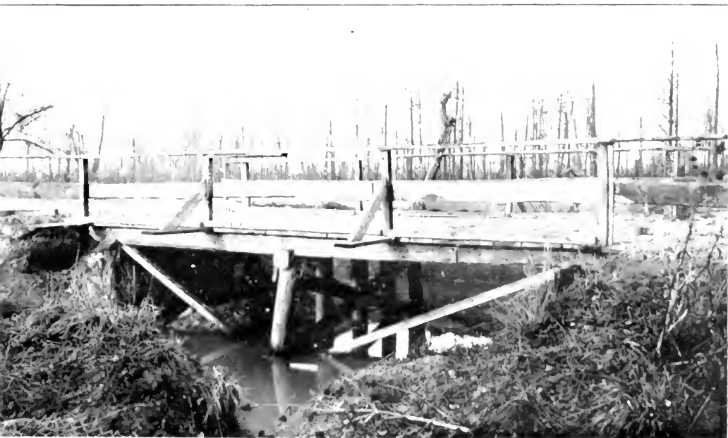
BRIDGE BUILT BY COMPANY "F" IMMEDIATELY FOLLOWING THE GRANTING OF THE ARMISTICE TO FACILITATE FOLLOWING UP OF 10TH ARMY
