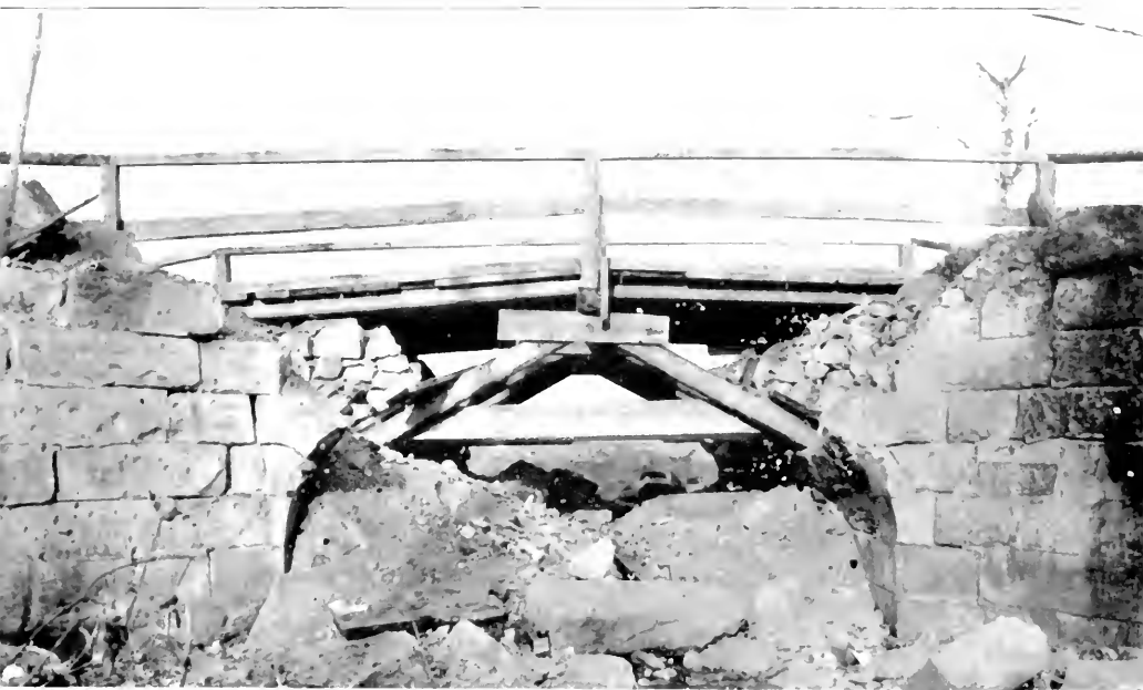
"A" TYPE BRIDGE CONSTRUCTED BY "F" COMPANY NEAR RIADVILLE,
