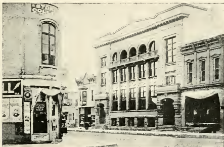
WISCONSIN STREET FRONT OF CITY HALL, PORTAGE
