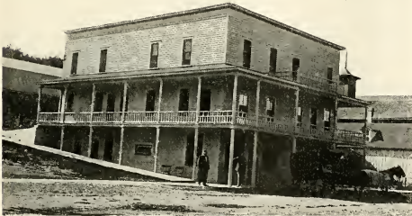
OLD CAMBRIA HOTEL (REMODELED)
