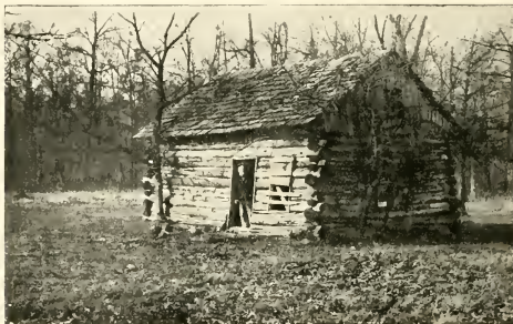
LOG CABIN OF THE REAL SETTLER
