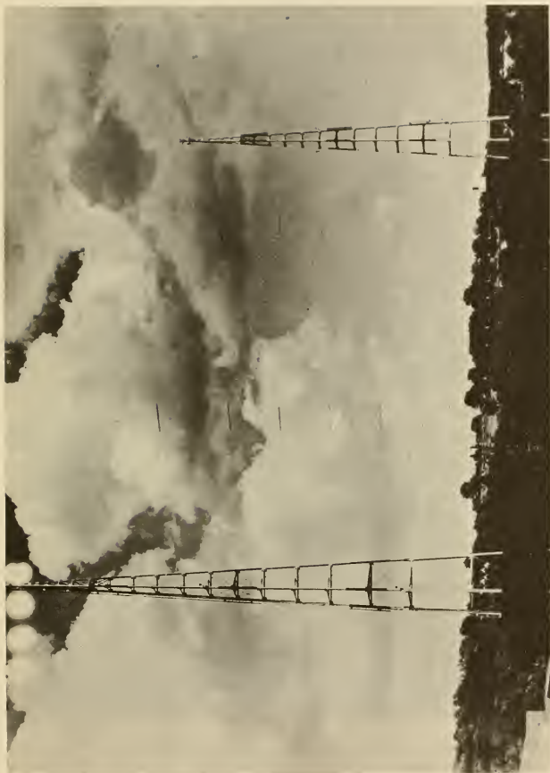
FIGURE 38-1. 28 Megacycle radar antenna used by U.S. Naval Research Laboratory for detection of aircraft by beat method in 1930, and for radar (pulse technique) in 1936.
