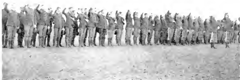
SWEARING IN COMPANY K, AT NIANTIC, TUESDAY, MAY 17, 1898.
