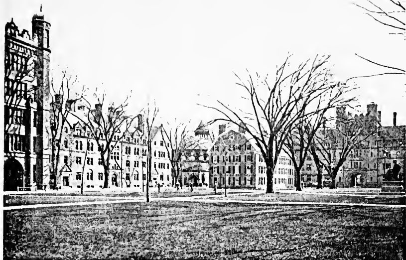
The Buildings of Modern Yale University: Phelps Gateway and Hall at the Left, then Welch, Osborn, and Vanderbilt; with "Old South Middle," now Connecticut Hall, near the Center, and President Woolsey's Statue at the Right of it
