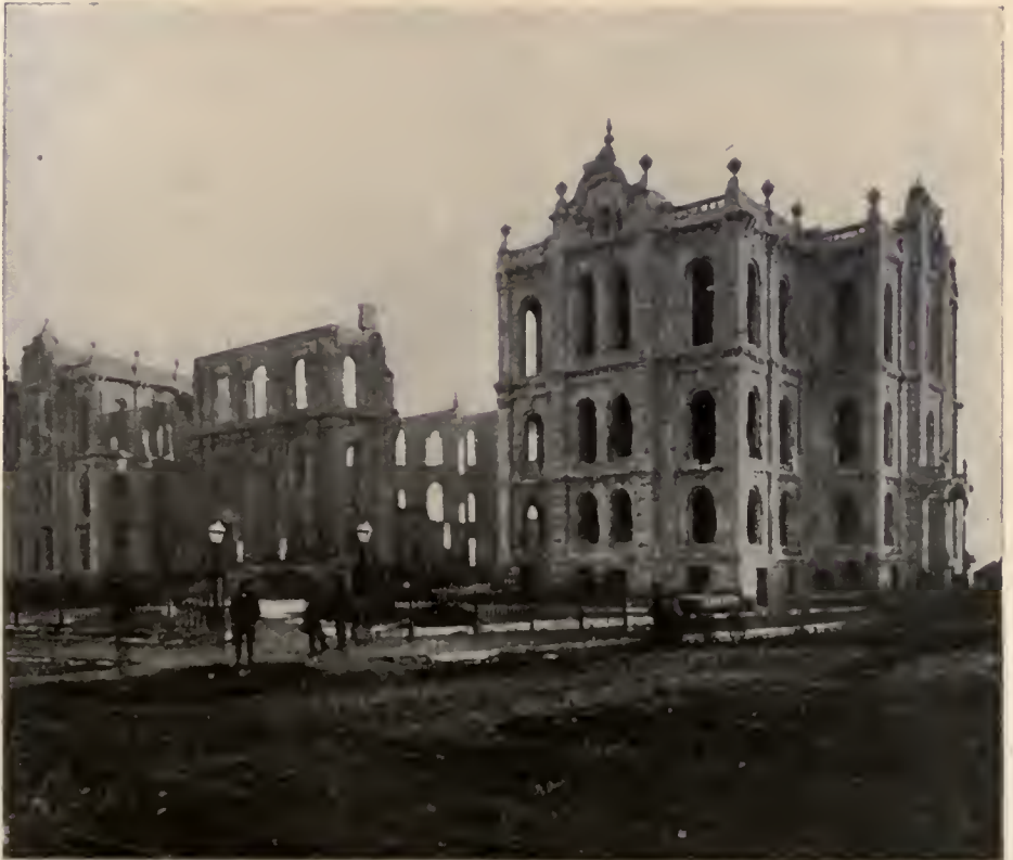
FOURTH COURTHOUSE. RUINS OF THE 1871 FIRE.
