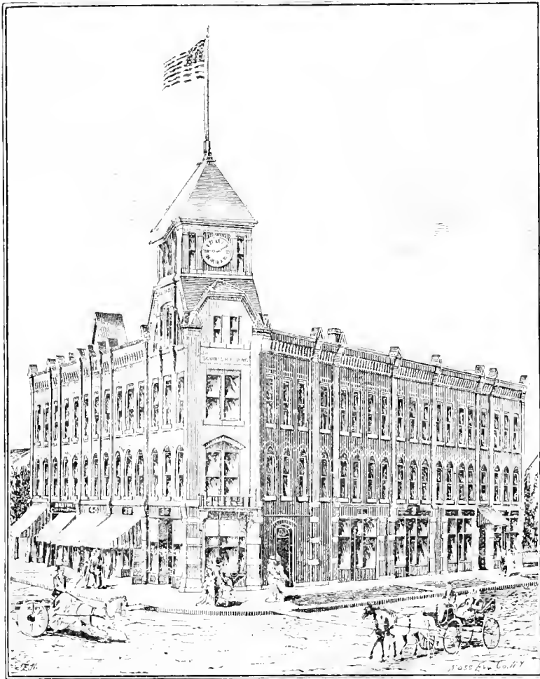
THE SQUIRES BUILDING, CORTLAND, N. Y.
