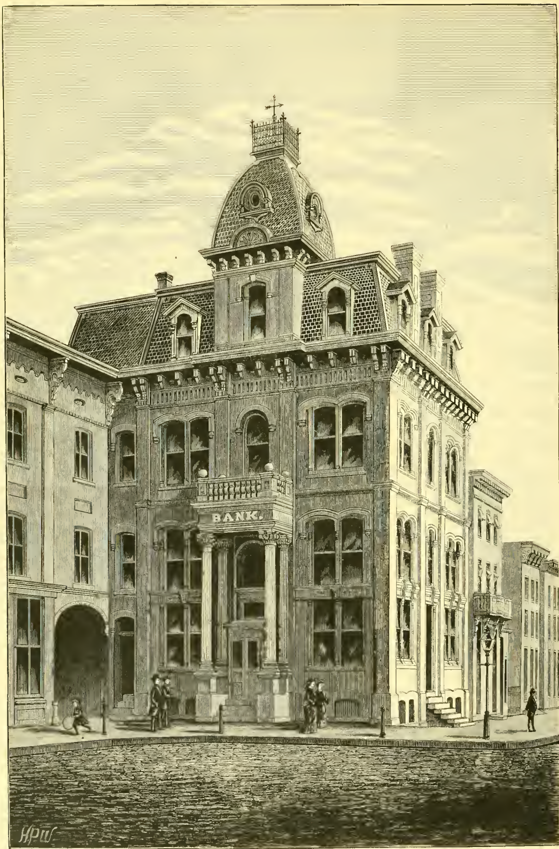
SECOND NATIONAL BANK BUILDING, ALLENTOWN, PA.
