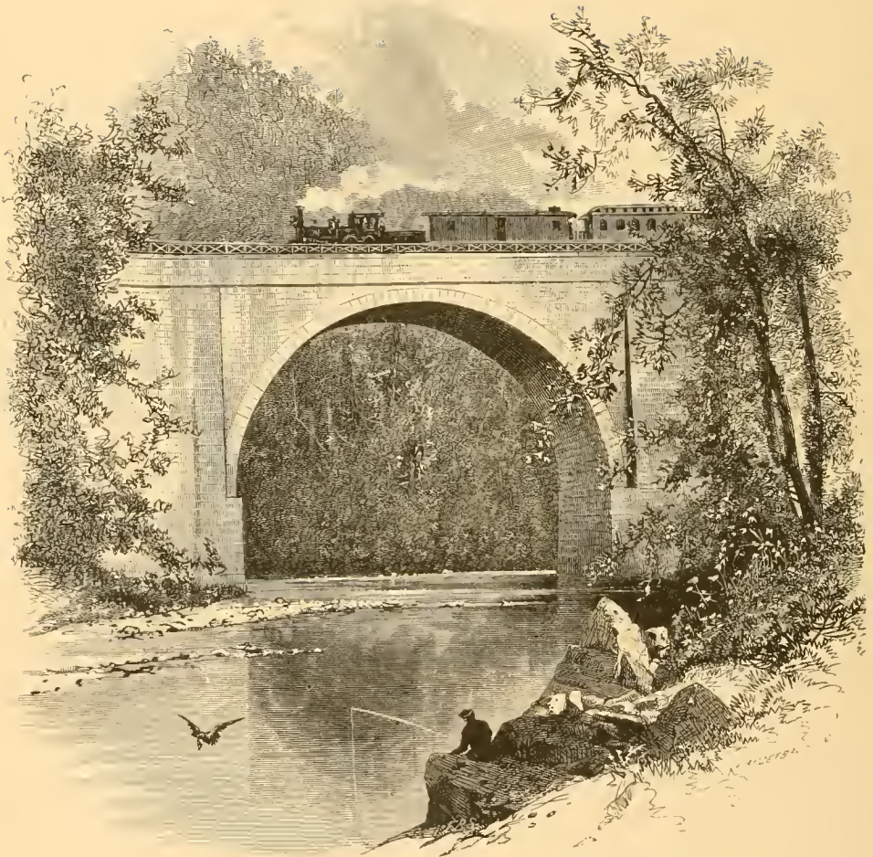
GONEMAUGH VIADUCT ON PENNSYLVANIA RAILROAD.
