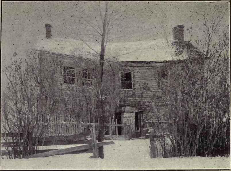
ARCHIBALD MCNEIL RESIDENCE, CLARKVILLE.
