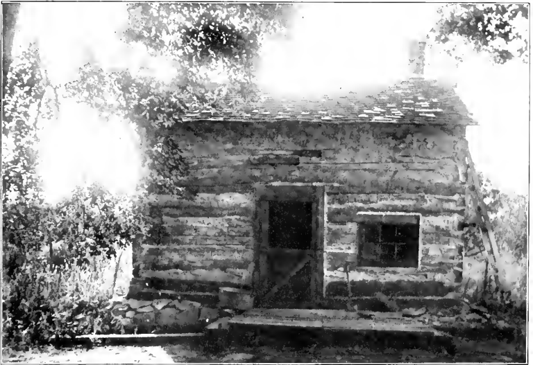
THE TEFT CABIN NEAR STENNETT—The only one extant in the western half of county. A survival of the fittest and exceptional because constructed of hewn logs.
