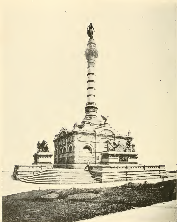
VIEW OF MONUMENT FROM SOUTHWEST.
