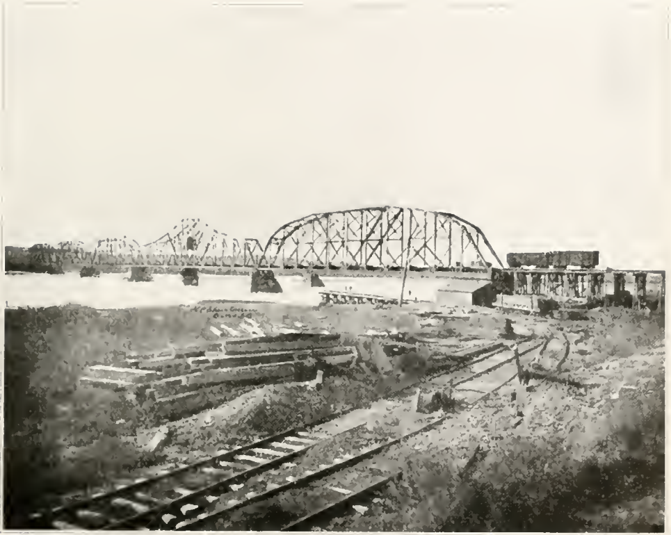
NORTHWESTERN RAILROAD BRIDGE AT PIERRE
