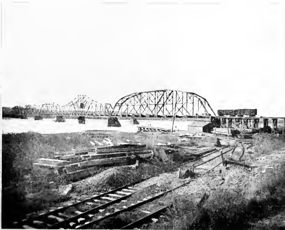
NORTHWESTERN RAILROAD BRIDGE AT PIERRE
