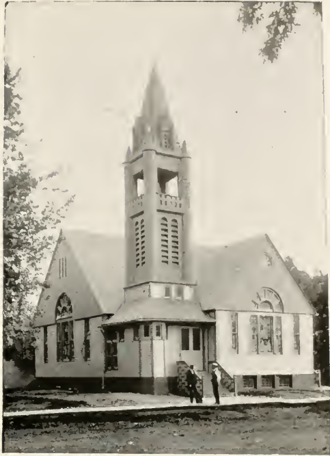
METHODIST EPISCOPAL CHURCH, GARDEN GROVE
