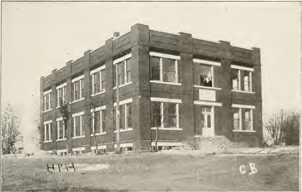
THE PRESENT HERALD BUILDING Erected in 1907
