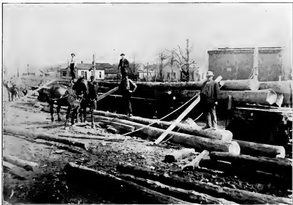
DOUBLE LOAD OF PILES, 78 FEET LONG, CUT IN DECATUR COUNTY BY T. E. DAY AND LOADED AT NEWPOINT, FOR USE BY THE BIG FOUR RAILROAD AFTER THE GREAT FLOOD OF 1913.
