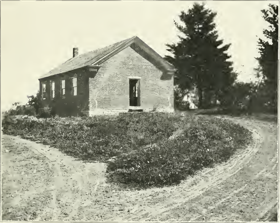
FIRST SCHOOL BUILDING IN COLESBURG
