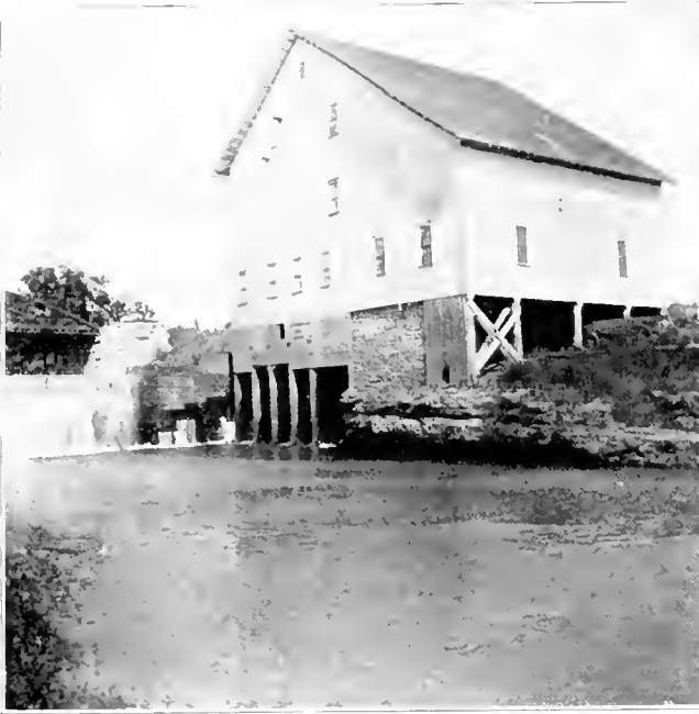
OLD QUAKER MILL, NOW MANCHESTER FLOUR MILLS, TWO AND ONE-HALF MILES NORTHWEST OF MANCHESTER.
