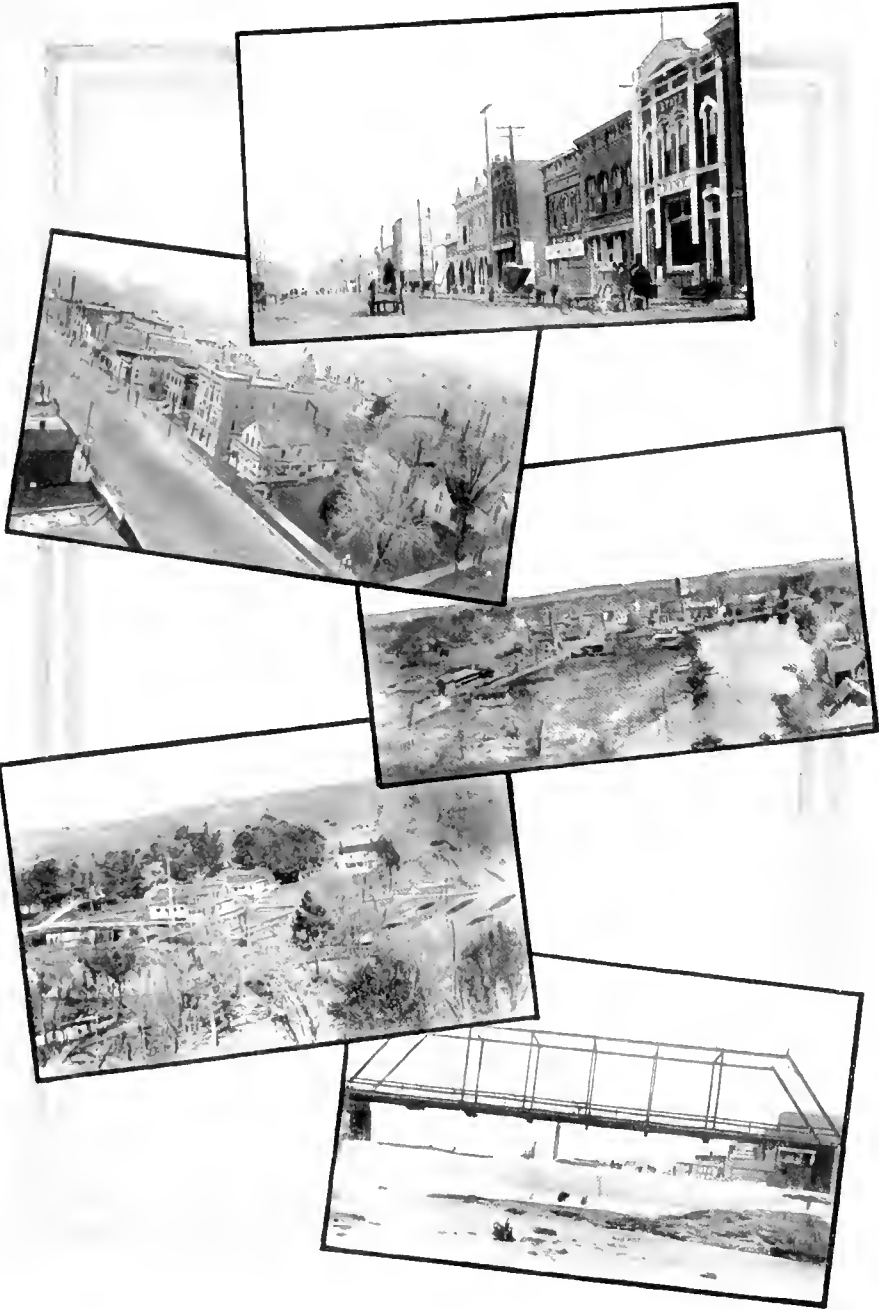
Bird's eye View from Courthouse.
