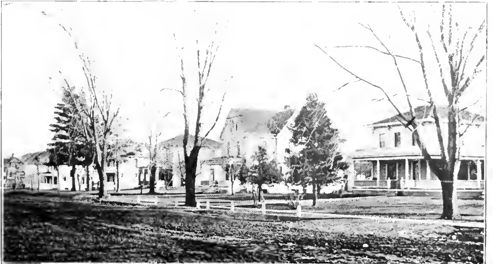
RESIDENCE VIEW, MEDIAPOLIS
