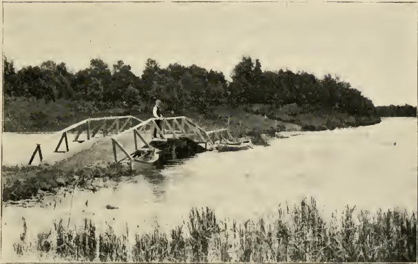
BRIDGE BETWEEN MINNIE WASHTA AND GAR LAKE.
