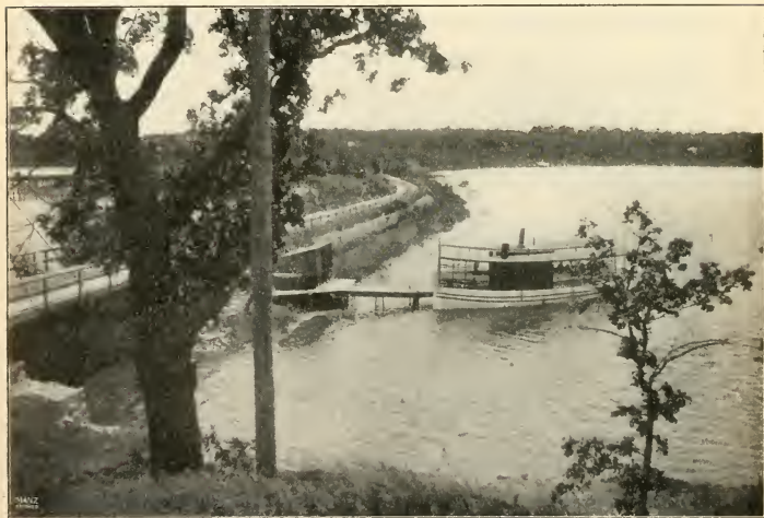
OKOBOJI BRIDGE AND GRADE LOOKING NORTH.
