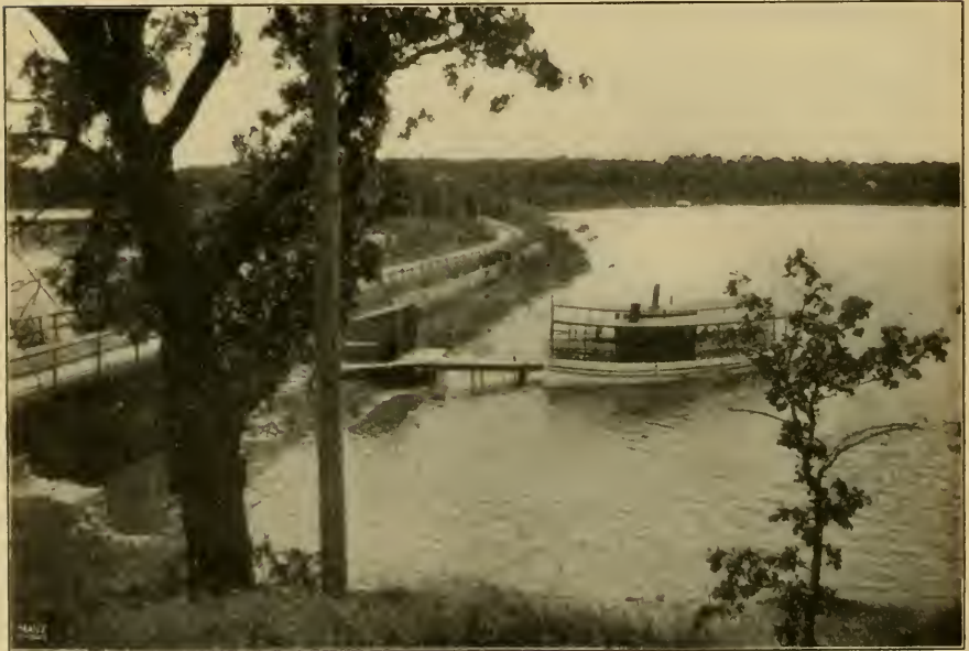
OKOBOJI BRIDGE AND GRADE LOOKING NORTH.
