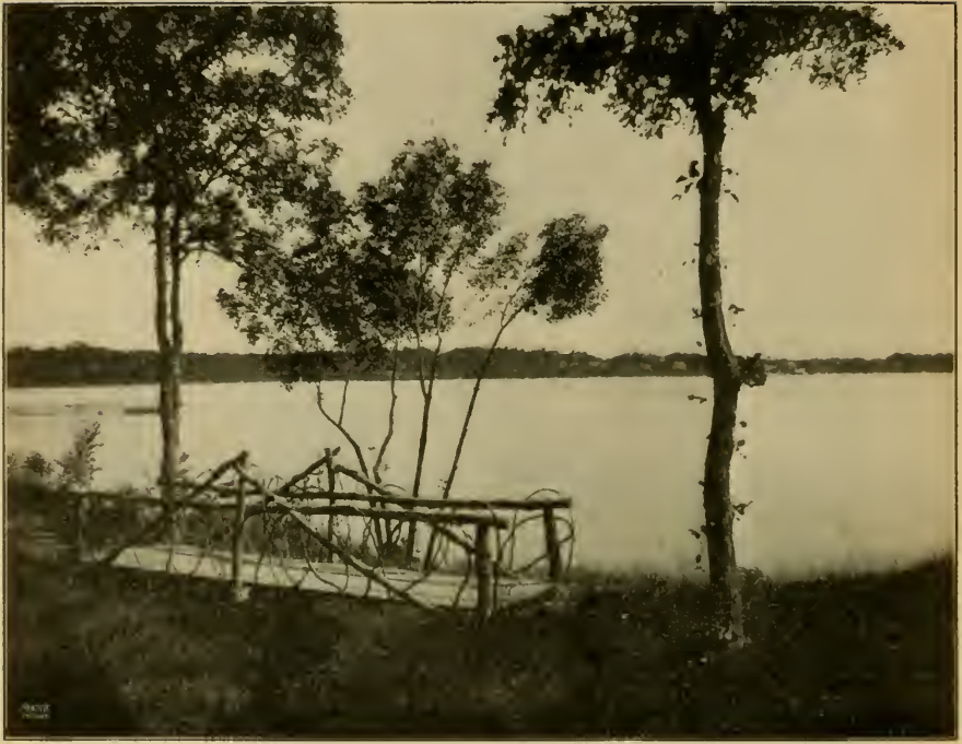
RUSTIC BRIDGE — DES MOINES BEACH IN DISTANCE — LOOKING EAST.
